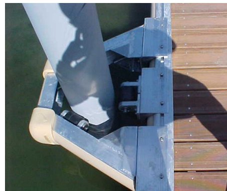
Image 2. Fixing the pontoon terminal with steel piles
